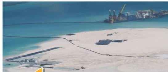
Johnson South Reef Military structure, Feb 2014
